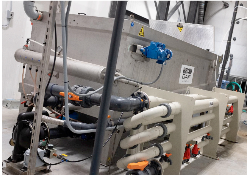
ALPHA 20 DAF and Pipe Flocculator
