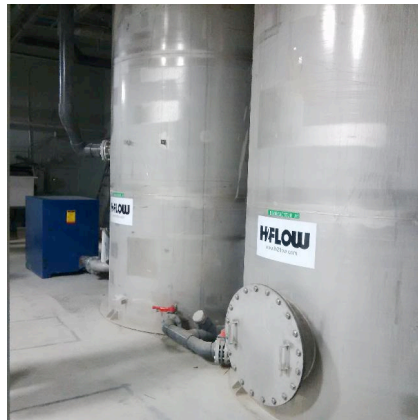
BIOWATER CMFF Bioreactor Units and Blowers
